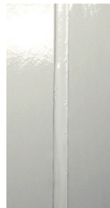
Polyurathane Seam Sealant
